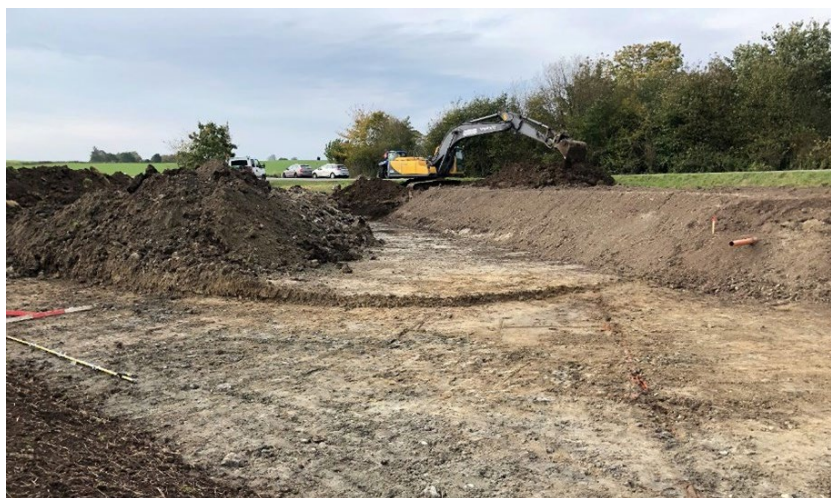
Above: Constructed wetland being constructed. October 2020. Photo Credit: SEGES
